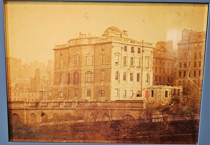
This photograph from 1865 shows the early stages of the transformation. Work has just commenced on one of the two new wings. This window, highlighted in red, has already been obscured. The Bank's staff continued working inside the building throughout the entire process.
